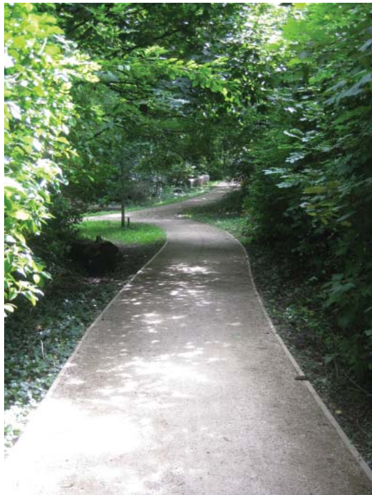
COMPACTED BALLYLUSK GRAVEL TREATED SOFTWOOD TIMBER EDGE
