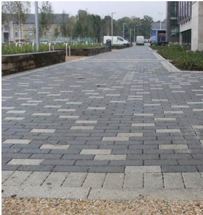
PCC MODULAR PAVING PERMEABLE 80mm deep
